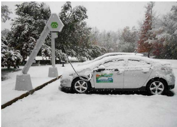
Figure 3.7: Retractable Cable for EVSE
