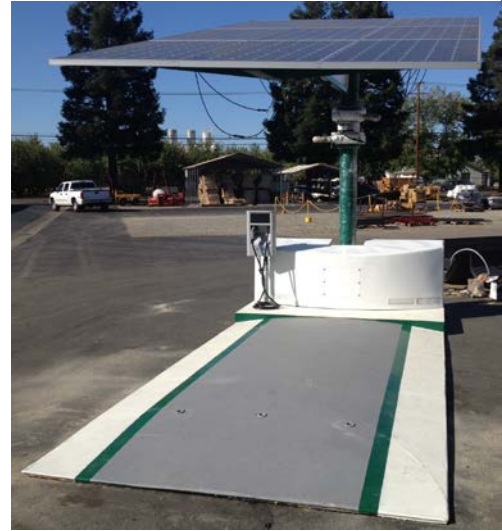
Figure 3.6: Solar Photovoltaic EV Charging Canopy
